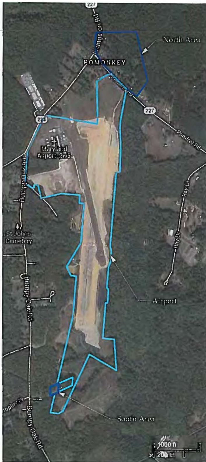
Figure 14. 2013 Aerial View Of Airport Area.
